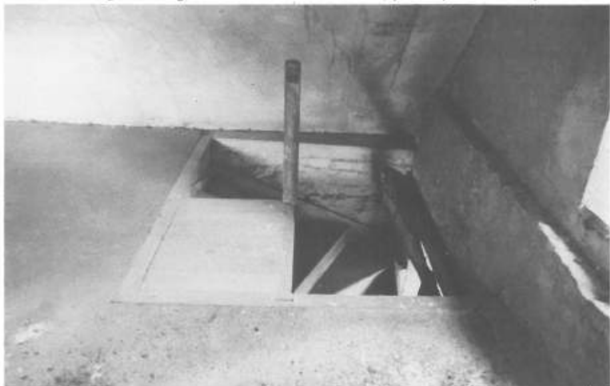
Head of timber stairs giving access to the attic storey.
