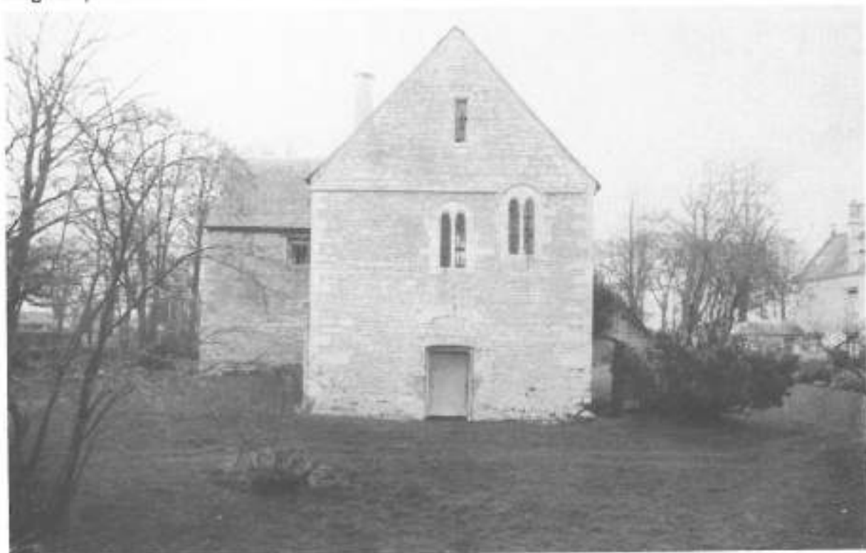
South elevation showing original (left) and added (right) south windows, and relieving arch of original window, replaced by modern door.
