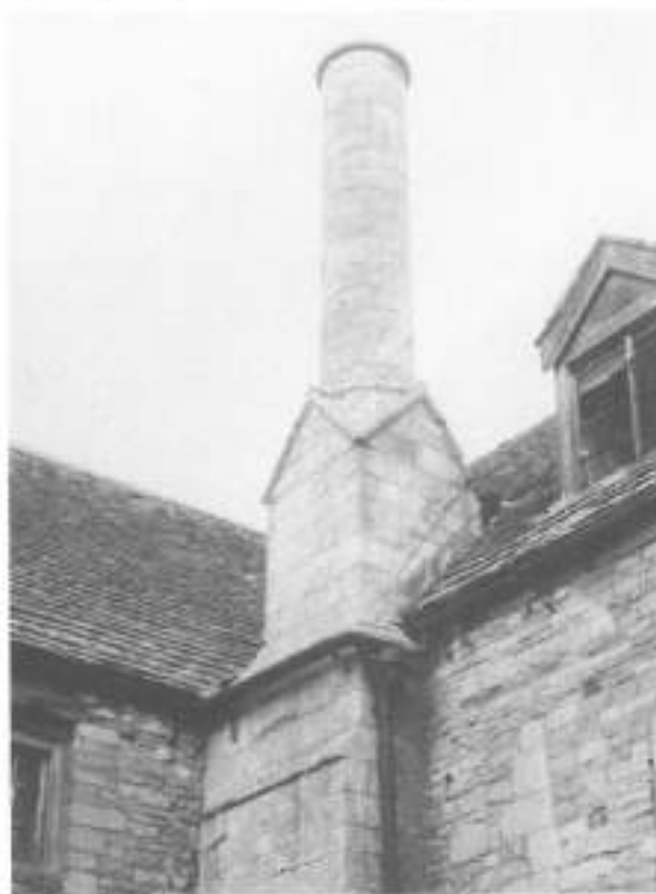
Detail of chimney, showing earlier, steeper, roofline.
