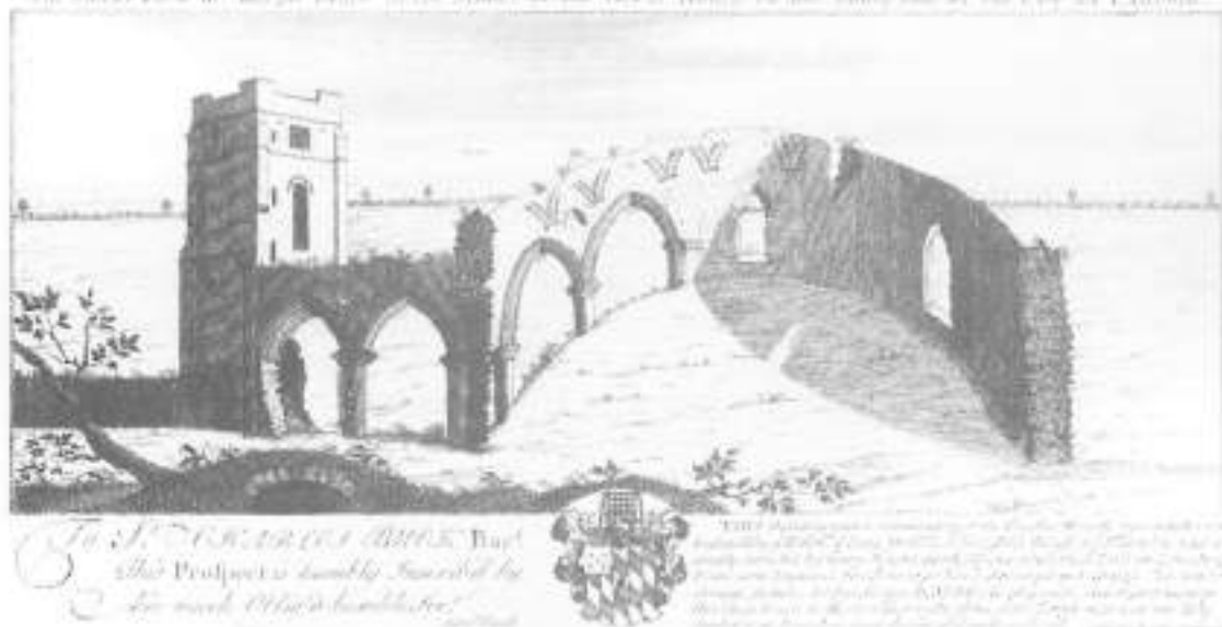
North view of Temple Bruer by Samuel Buck, 1726. This is the only illustration of the round nave to survive.
