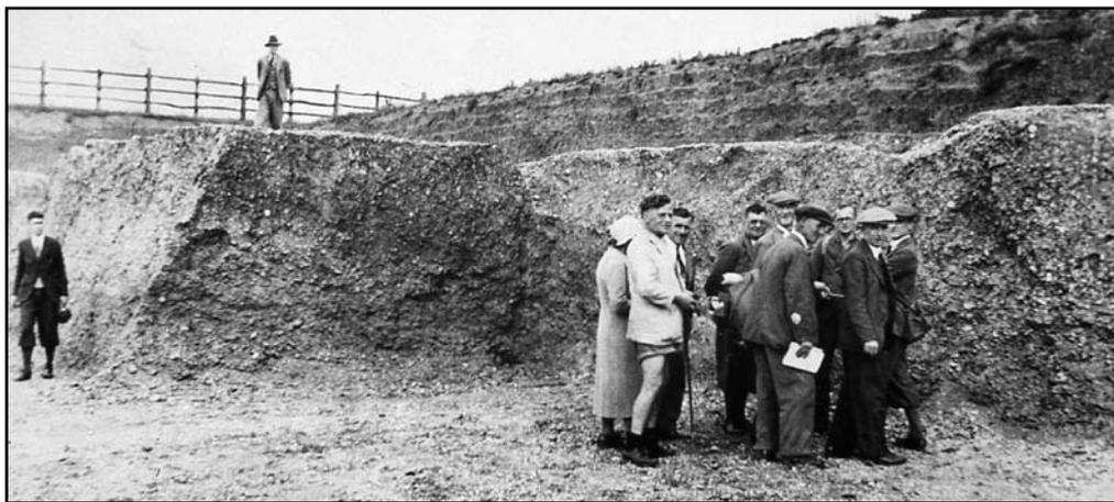
**Figure 2.** Kirmington gravel pit during the 1936 visit by the Sorby Geological Society. The section revealed 2.5m of flint beach shingle, overlain by 2m of reddish-brown till. View NE at TA104117. (Photo: AC Dalton.)
